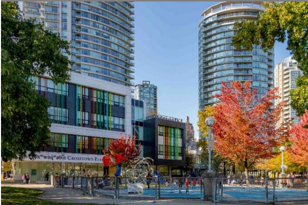
Crosstown ʘxʷwəqʷəθət Elementary School, Vancouver
